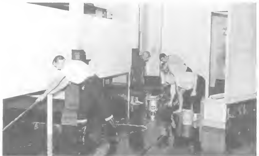
Attendants mopping up storm water in the main gallery in the 1960s.
